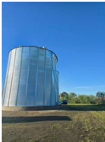
Damaged bins and sheds
